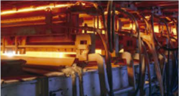
White hot ducts: Making mineral wool at the speed of sound
